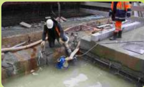
Dewatering Foundation, Trenches and Pits
